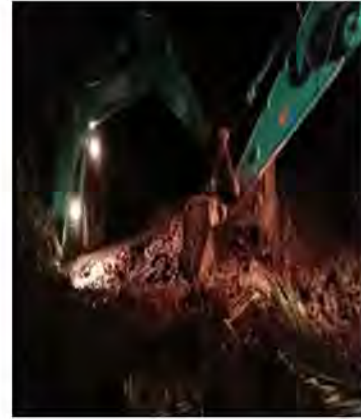
BANTUAN EXCAVATOR Excavator Assistance
